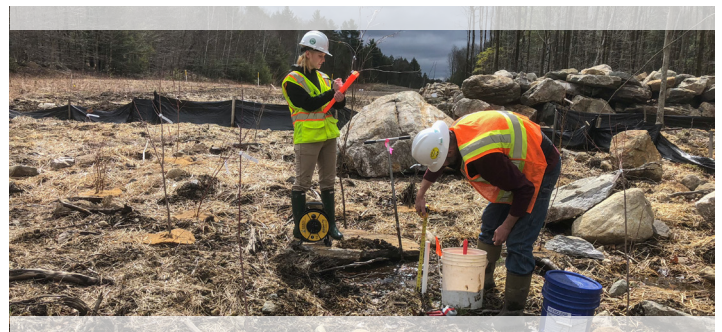
Post construction vegetation planting - installing ground water monitoring wells
